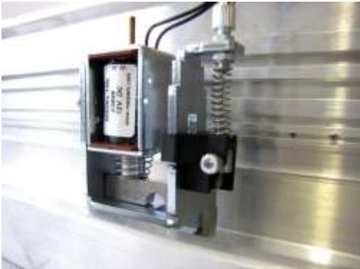
Check that the manual release works, when the knob is in the locked position, the electric lock must work normally.
