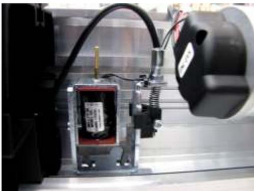
In case of single-leaf installation, the electric lock must be installed at one end of the transom.
