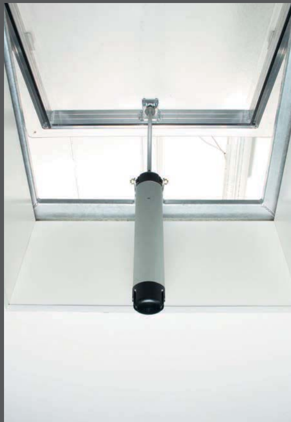
Installation on dome with fixing end brackets
