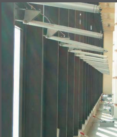
Installation on top hinged window with connection to compressed air system
